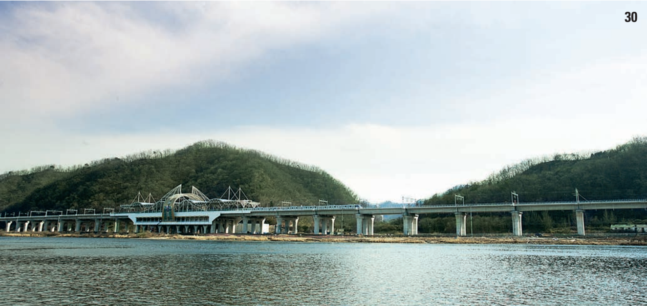
29. Expressway No. 45 (Hyeonpung-Gimcheon Section) Location: Gimcheon, Korea - Total Length: 28.8km, 4 Lanes - 32 Bridges (6.05km) - 4 Tunnels (7.7km) Project Period: 2001.12 ~ 2007.12 30. Electrified Double Track Railway in Gyeongchun Line Section No. 7 Location: Chuncheon, Korea - Total Length: 12.15km, 5 Bridges (3.22km) - 4 Tunnels (8.19km), 2 Stations Project Period: 1999.12 ~ 2011.12
