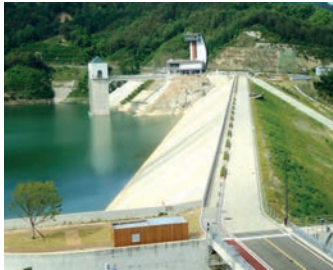
Renewable (Pumped Storage Hydroelectricity)
