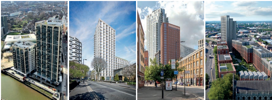
CREEKSIDE, GREENWICH ADDISCOMBE GROVE, CROYDON EAST ROAD, LONDON CAMP HILL, BIRMINGHAM
